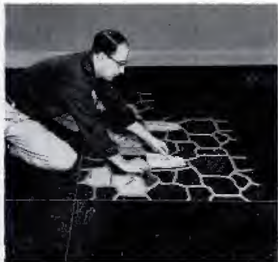
Grids are laid in place, then tiles fitted in. Tiles and grids in single carton will cover 54 square feet
